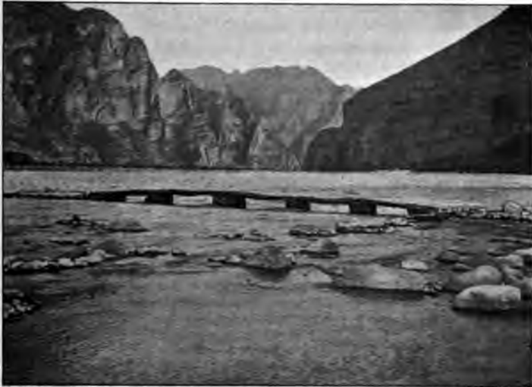
GORGES ON THE CHU-MA HO, WITH NATIVE BRIDGE.
